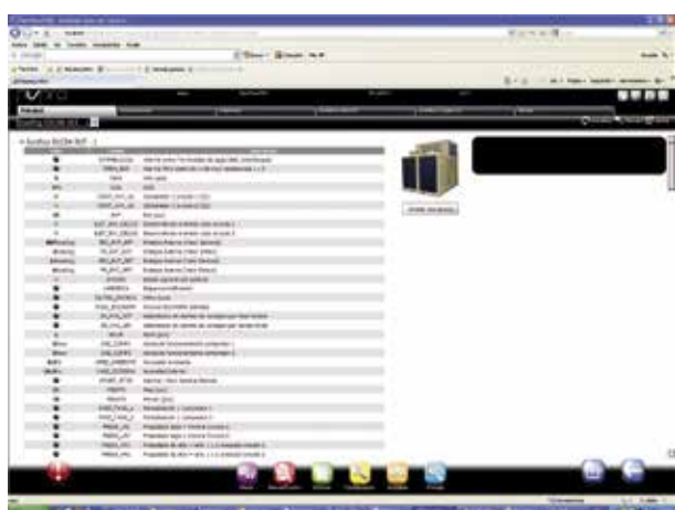
Rooftop detail screen: makes it possible to visualise and change all parameters via the PI@nt Visor.
